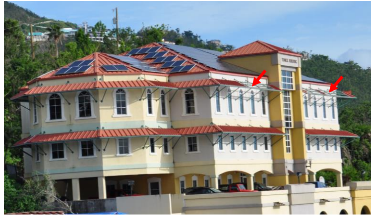
Figure 2. A relatively large PV array on a commercial building. Several metal roof panels were blown off the overhang (red arrows), but there was no apparent damage to the array.
