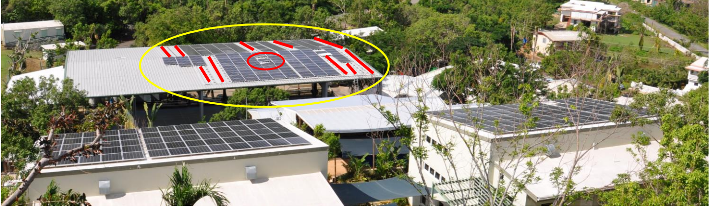
Figure 5. Roof where several adjacent panels were blown off (red lines). See Figure 6 for the area within the red oval. There was no apparent damage at the PV array at the lower left building. The array at the lower right building may have lost a panel or two.
