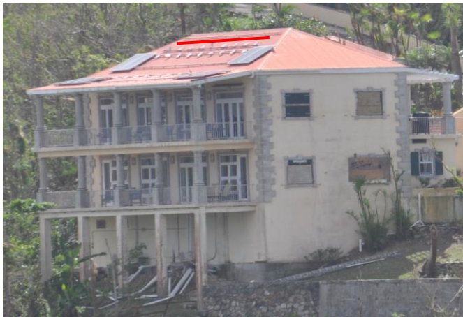
Figure 3. All the PV panels in the top row (red line) were blown off. Most of the panels in the middle and bottom rows were also blown away at this residence. All the panels detached from the rails.
